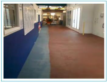
Due to the nature of the works that take place within the facility, the client requested areas to be demarcated to maintain a safe working environment. This was achieved in the first instance by the installation of different colours of our Stonclad GS mortar.
