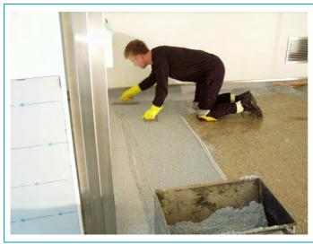
Installation of Stonblend GSI at 6mm thick with 150mm high coves.
